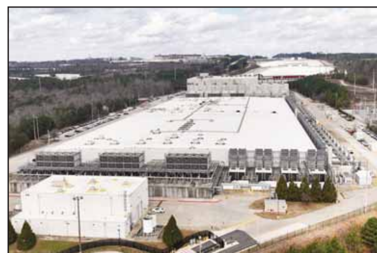
The Douglas County Google Data Center complex is visible, March 6, 2026, in Lithia Springs, Ga. (AP)
